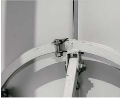
Assemble the LNB mount as per pictures. Fit LNB tubes protruding 37mm and tighten all clamps. Fit to dish LNB support rods including the C Band brackets. Do not fully tighten support rod bolts at this stage.
