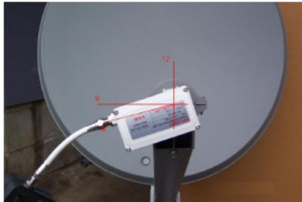
**Step 3:** Set elevation (up and down angle of the dish) using scale or marks on the dish mounting bracket, to required angle as determined by the angle chart on our website or from your own calculations.
